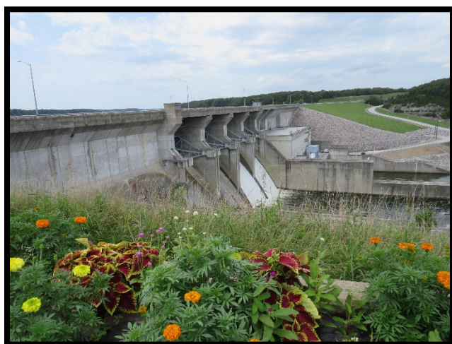
Figure 5-16. Warren G. See South Spillway Overlook
